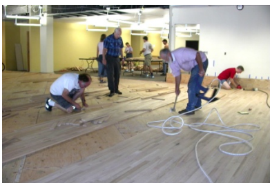
Nailing the ballroom floor
