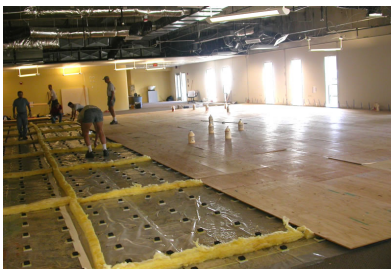
Ballroom floor in progress
