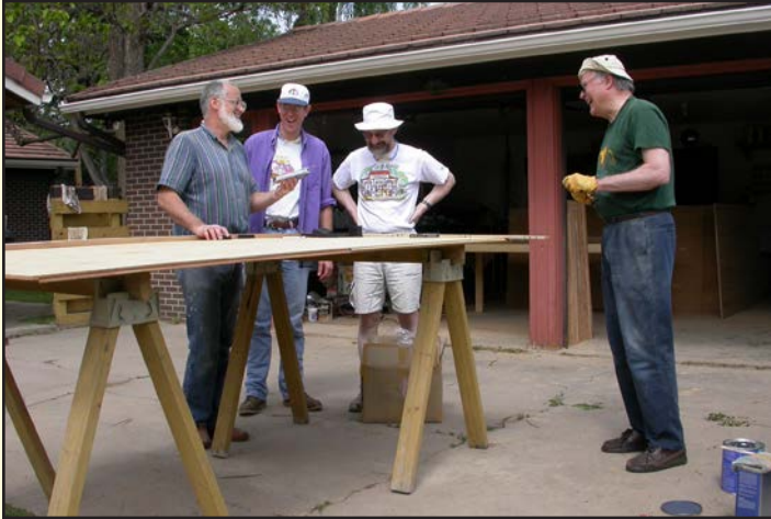
Phil Rice, Jerry Olson, Rod Frehlich and Dan Anderson joined the volunteer crew building the new floor.
